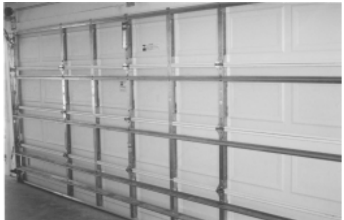
Garage Door Bracing (Opening Protection)
