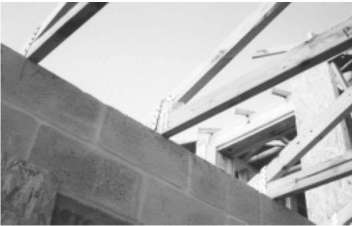
Hurricane Straps (Roof to Wall Connection) and Masonry Wall Construction
